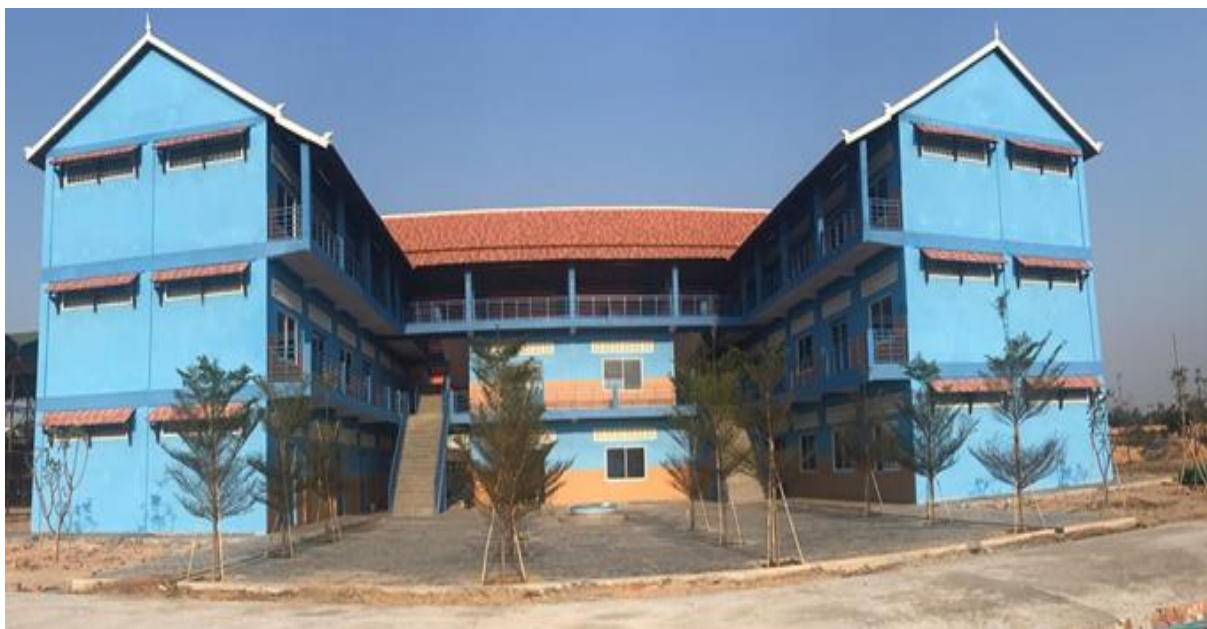
Completion of the new St François Technical Campus
