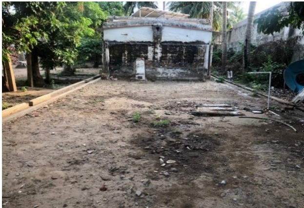
Site clearance - April 2017
