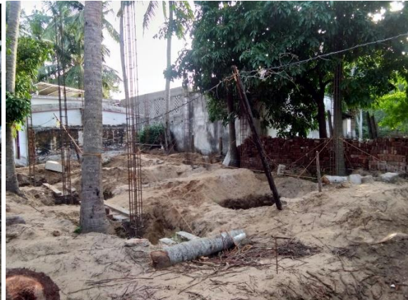
Foundations for construction begin - May 2018
